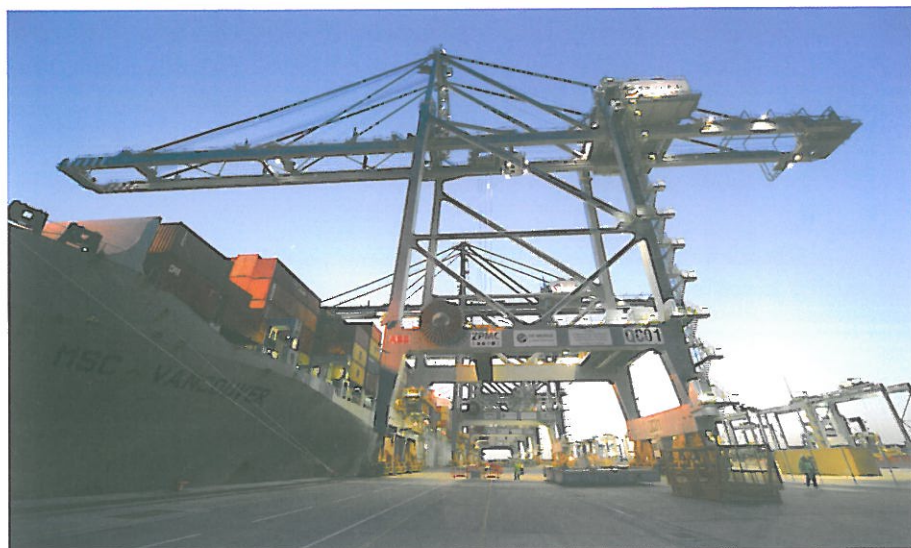
Container cranes are growing in size as ships get bigger
